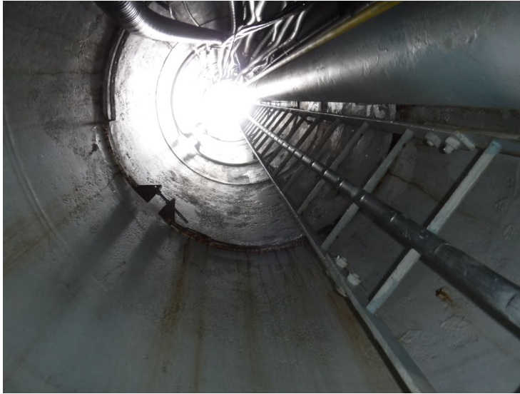
31) Spot coating failures in the access tube.
