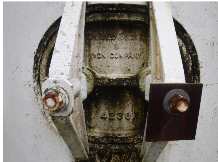
5) The original riser manway is in good condition.
