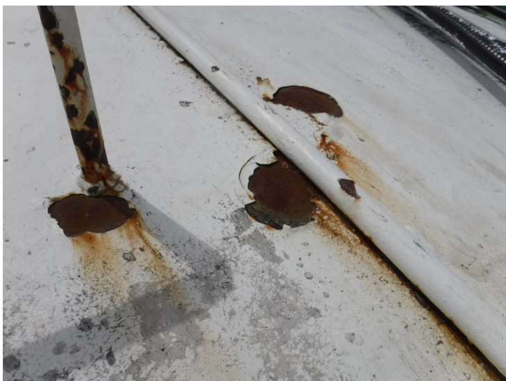
21) Spot coating failures on the outside of the handrail.
