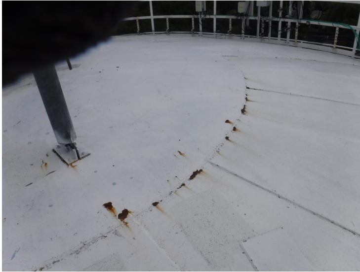
19) Spot coating failures on the roof inside the handrail.
