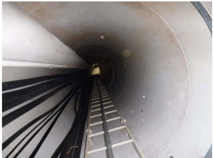
29) The access leg coating is in good condition overall.
