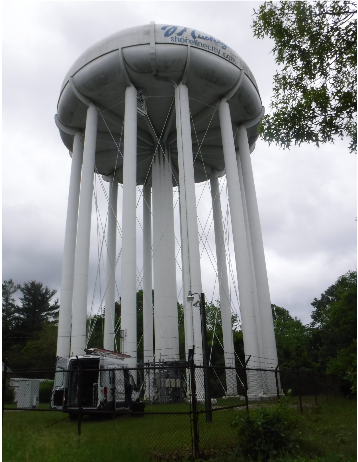
1,000,000 gallon radial arm tank (Marshall) located in Muskegon, Michigan.
