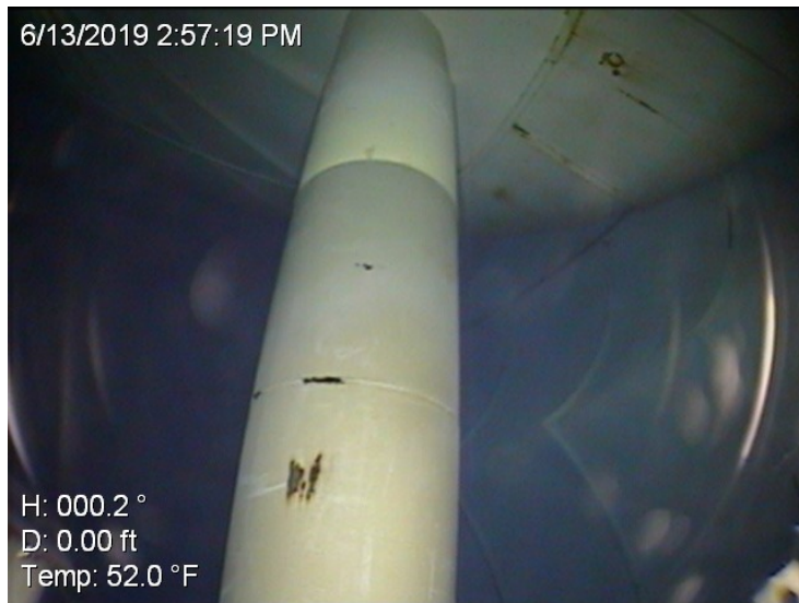
49) Spot coating failures on the access tube below the high-water line.
