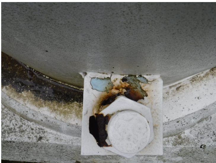
9) Coating delamination and spot coating failures to the substrate on a leg anchor bolt.
