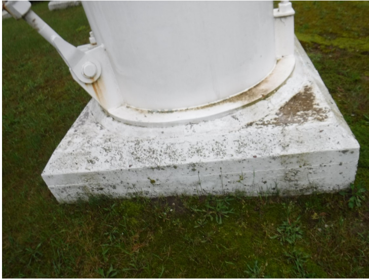
7) Typical leg foundation is in good condition.
