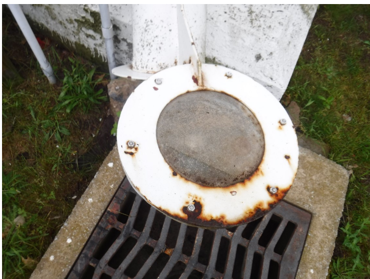
12) The screen on the overflow flap gate is in good condition.
