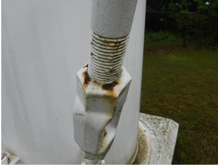
10) Spot coating failures on a sway rod turnbuckle.
