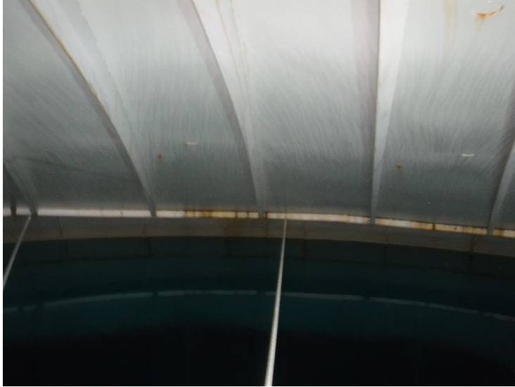
37) The roof coating is in good condition overall.
