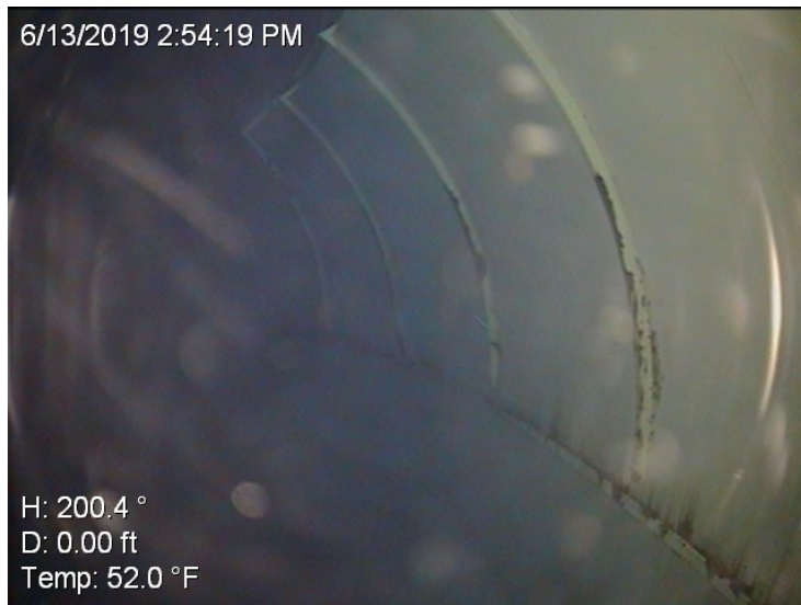
40) Coating failures on the roof knuckle stiffeners.
