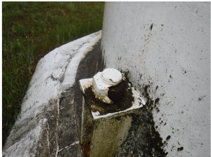
2) Corrosion on a riser anchor bolt.
