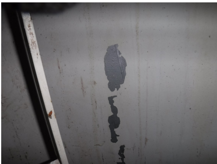
30) Coating delamination on the access leg exposing the previous aluminum coating.
