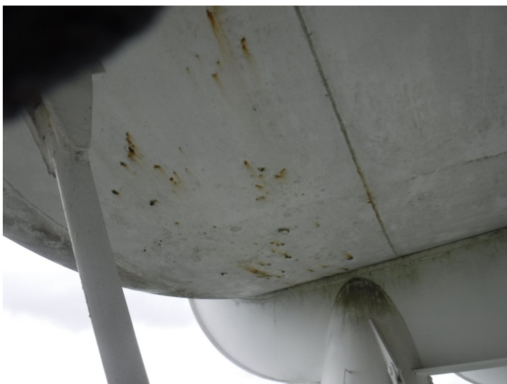
18) Spot coating failures on the bowl.
