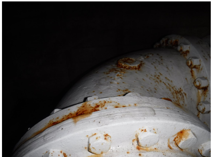
53) Rust bleedthrough mainly on the bolts and flanges.
