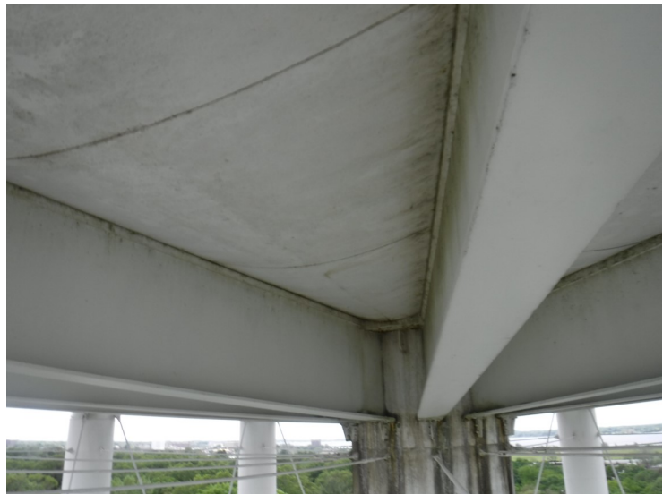
17) The bowl coating is in fair condition overall.
