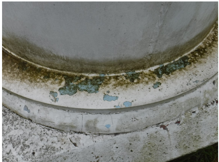
8) Coating delamination on a leg baseplate.
