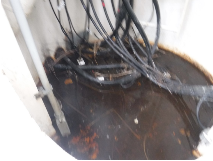
28) Water pooling on the access leg baseplate.
