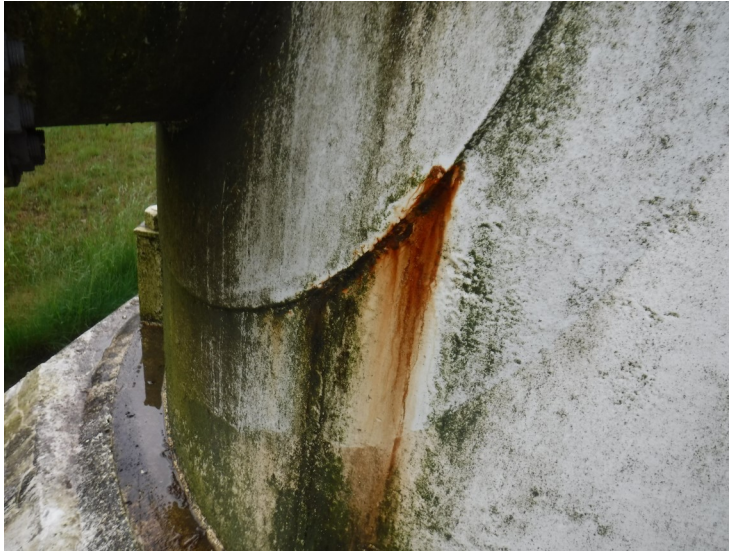
4) Spot coating failures on the riser manway reinforcement plate weld seam.
