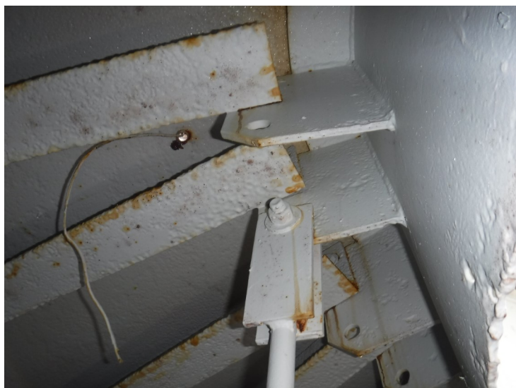
36) Corrosion at the roof stiffener edges.
