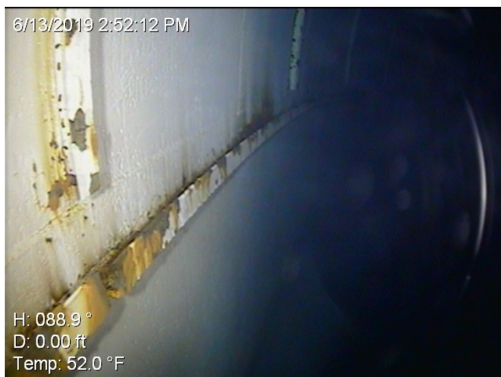
42) Coating failures on the sidewall stiffener.
