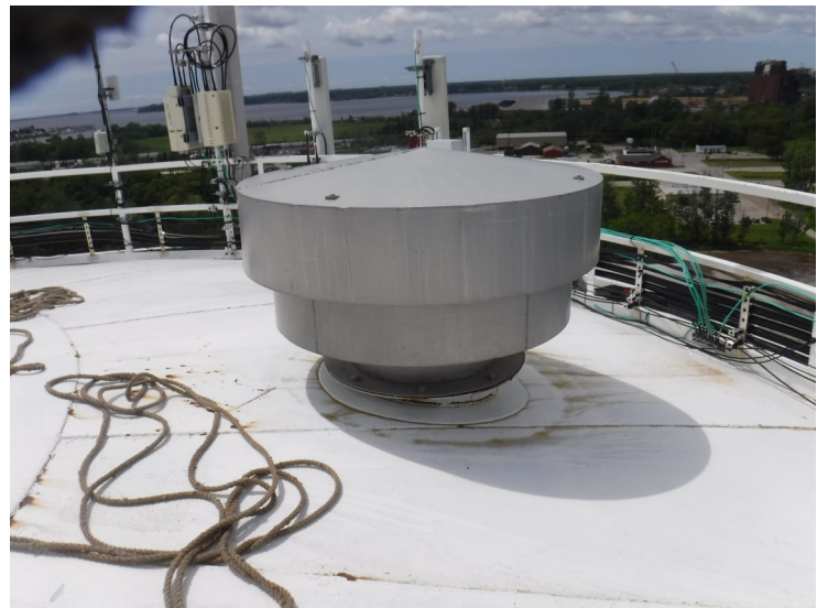
23) The frost-free roof vent is in good condition.
