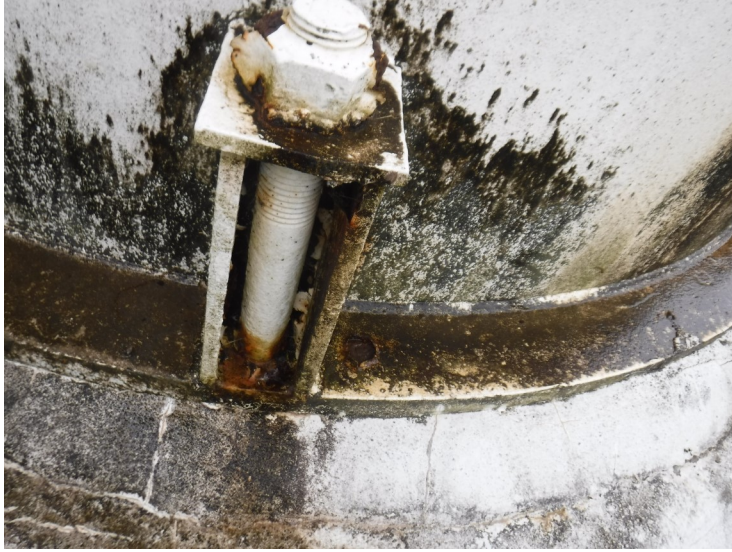
1) The riser foundation and anchor bolts are in good condition. There are cracks in the tapered grout.
