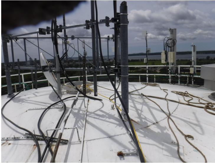
25) There is an antenna mounting structure on the roof and the handrail is also being used for antenna mounting.
