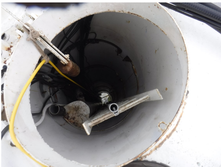
33) The access tube location is outside the handrail.
