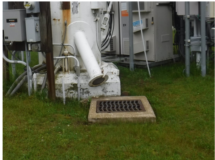
11) The overflow pipe discharges to a catch basin.
