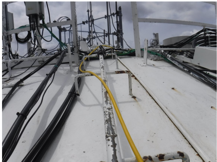
26) Spot coating failures on the roof ladder rungs from the access tube to the center of the tank.
