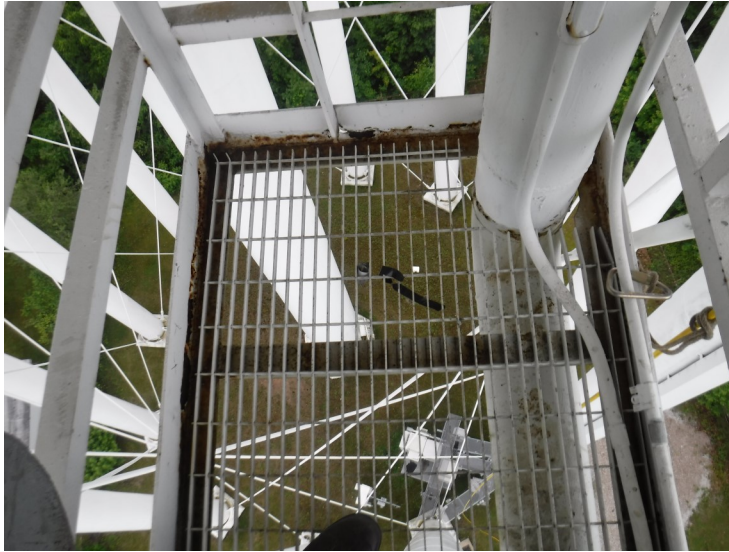
16) The catwalk from the leg to the access tube is in good condition.
