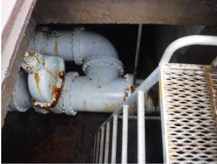
52) The piping located in an adjacent pit is in good condition.
